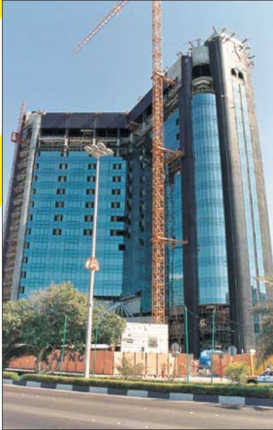
SHAIKH FATMA TWIN TOWER - ABU DHABI
